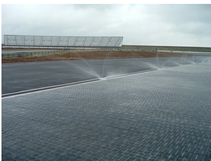
Skidpan Rockingham Speedway Northamptonshire, Great Britain 270 Meter of MEADRAIN Supreme EN3000 with F900 gratings
