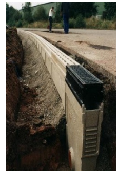
Dunlop test circuit – Wittlich-Neuerburg, Germany MEADRAIN Traffic D1000 with F900 gratings
