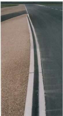
ATP test circuit – Papenburg, Germany (used a lot by Mercedes Benz) MEADRAIN Supreme EN1000
